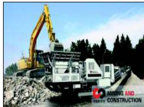
Figure 4: Mobile crusher fed by a loader.
