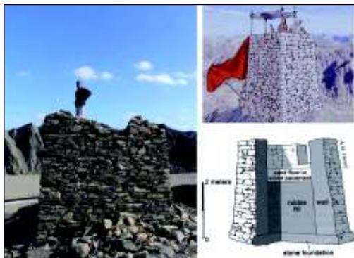
Figure 10. One of the best preserved signal towers: it is squared and built with slabs of the local schists (reconstructions from Sidebotham et al. 2008).
