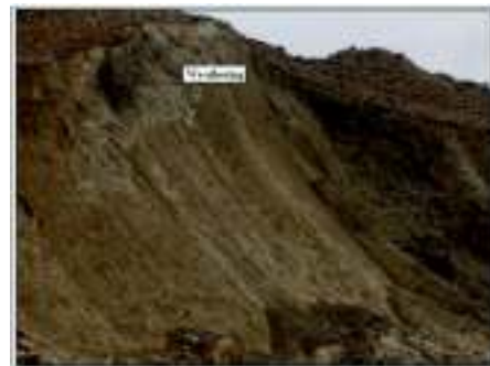
Figure 4. The failure surface of the Kef Essenoun landslide.
