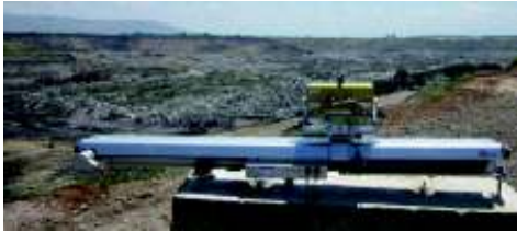
Figure 6. IBIS-M installation at Çollölar.
