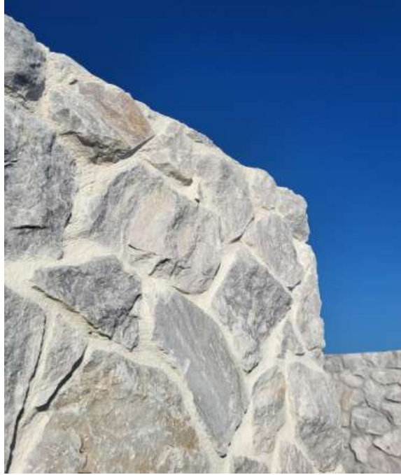
Figure 11. Scrap marble recovery
